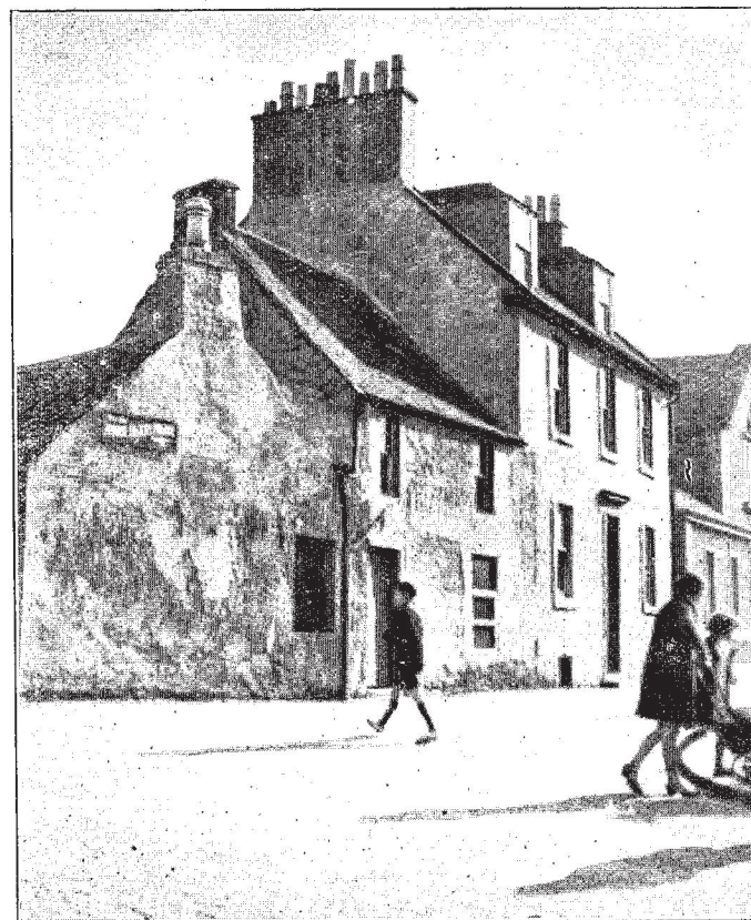
The larger of these buildings, situated at the corner of Stuart Street and High Street, was erected in 1628 and was known as the Drovers' Inn. The smaller building, known to many as Slaven's Fruit Mart, was removed in 1938, and in its place stands a replica of Rothesay's Old Mercat Cross.
